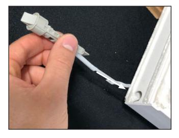
Install new replacement latch assembly by sliding into the latch pocket. Be sure latch assembly is flush with window stile.
