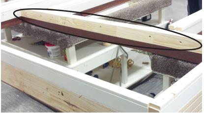
Remove 6-7 screws located on the bottom of the transom frame, connecting it to the door frame.
