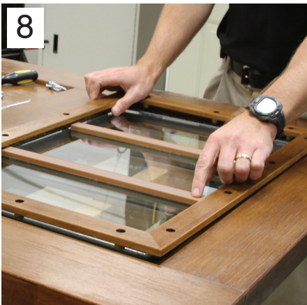
Step 8 Make sure interior and exterior trim are aligned with each other, then insert trim into door slab. Use a magnetic tip screw driver and make sure long screw bites into the exterior trim screw boss.
