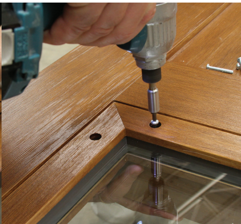
Step 8 Make sure interior and exterior trim are aligned with each other, then insert trim into door slab. Use a magnetic tip screw driver and make sure long screw bites into the exterior trim screw boss.
