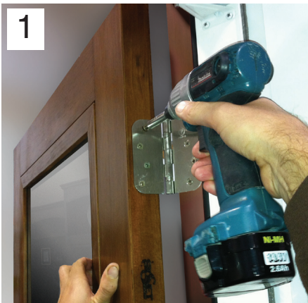
Step 1 Remove door slab from hinges.
