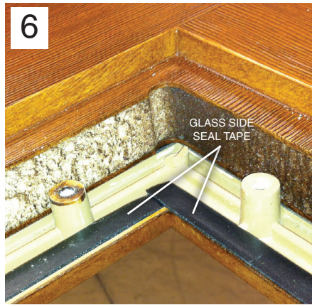
Step 6 Inspect glass side seal tape. If damaged, replace tape. If caulking is present instead of tape, remove and replace with new caulking.
