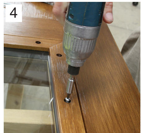
Step 4 Remove trim screws and trim.
